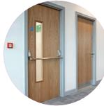
Emergency exit hardware to enable occupants to escape the building safely in an emgerency situation
