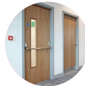
Emergency exit hardware to enable occupants to escape the building safely in an emergency situation
