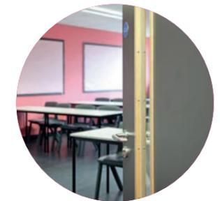
Light Reflective Value measurements can be supplied to provide the necessary colour contrast for BS 8300 compliance
