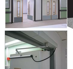
The door automation system was installed and commissioned by our team of Approved ADSA installation engineers to BS EN 16005. doors to be opened outwards by staff within just 15 seconds
